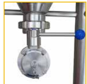
Butterfly valve for total drain
